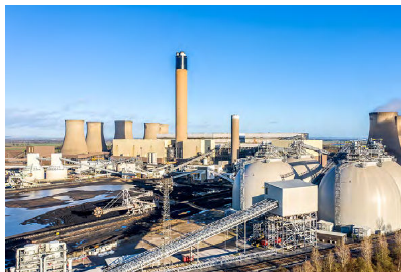
Drax Power Station, near Selby, North Yorkshire
